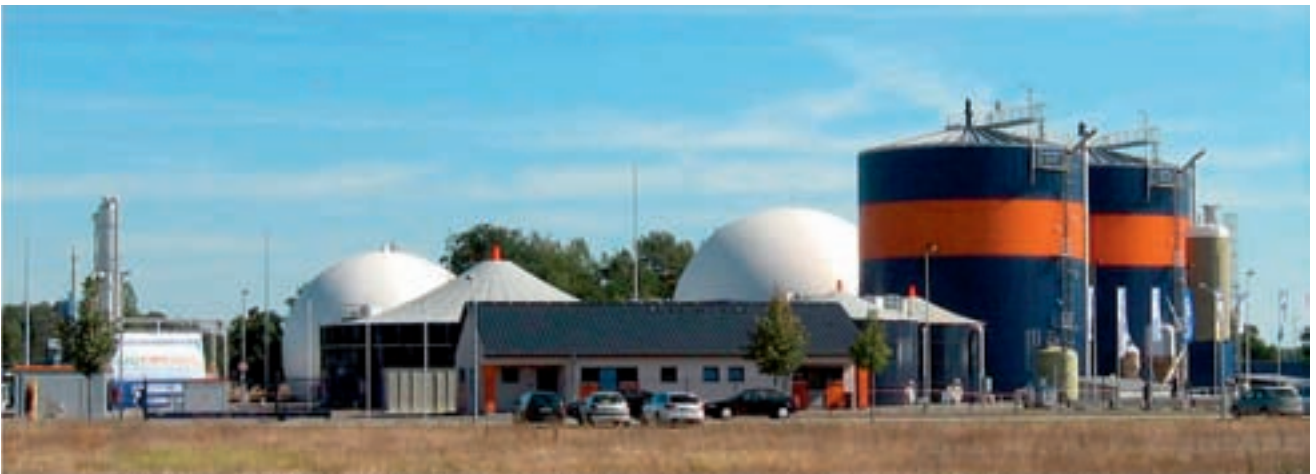
GreenGas Production site Rathenow
