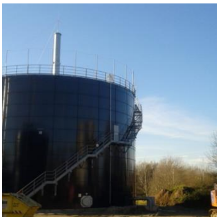
Bremen Seehausen treatment plant Low pressure gas depot 50 mbar Volume: 5,000 m 3
